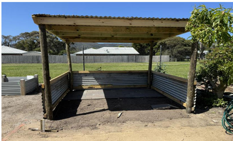
New Worm Farm under construction
