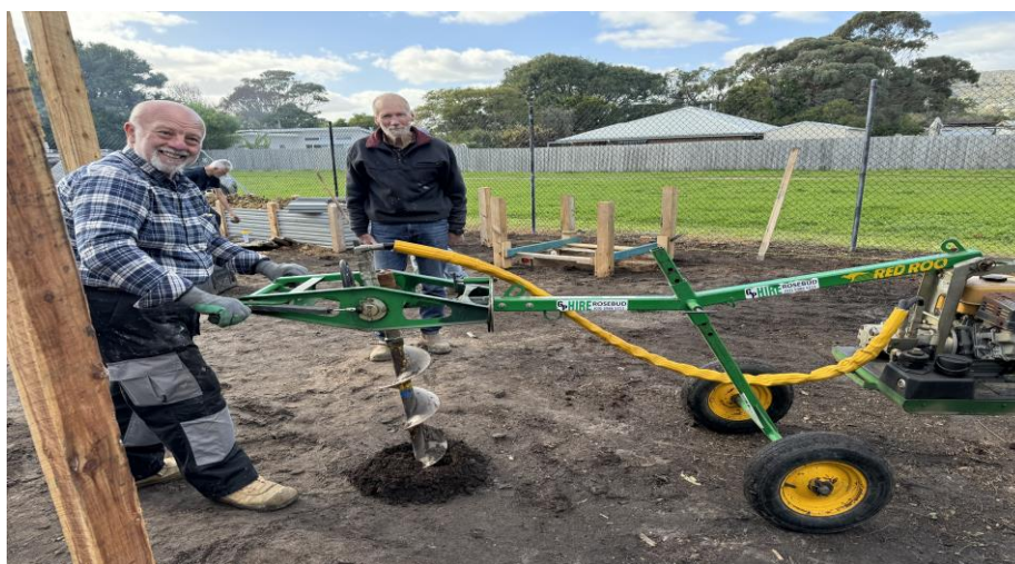
Sam and John digging postholes for the new shed.
